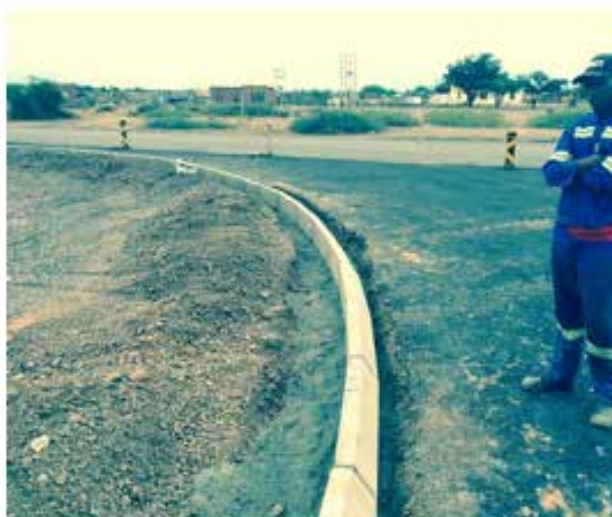
Installation of kerbs at intersection at km 0.000
