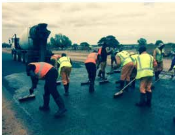
The 2 nd sub-contractor, Invula, applying slurry with a 7 m 3 mixer
