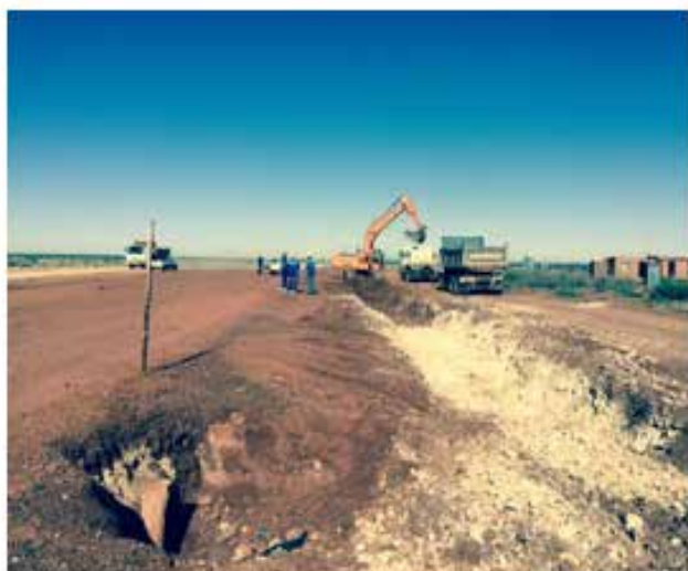
Excavating side drain at km 5.700 - km 5.800
