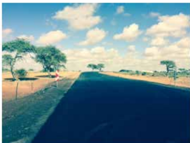
Installation of danger plates at culverts and 2 nd slurry on surfacing completed at km 0.100
